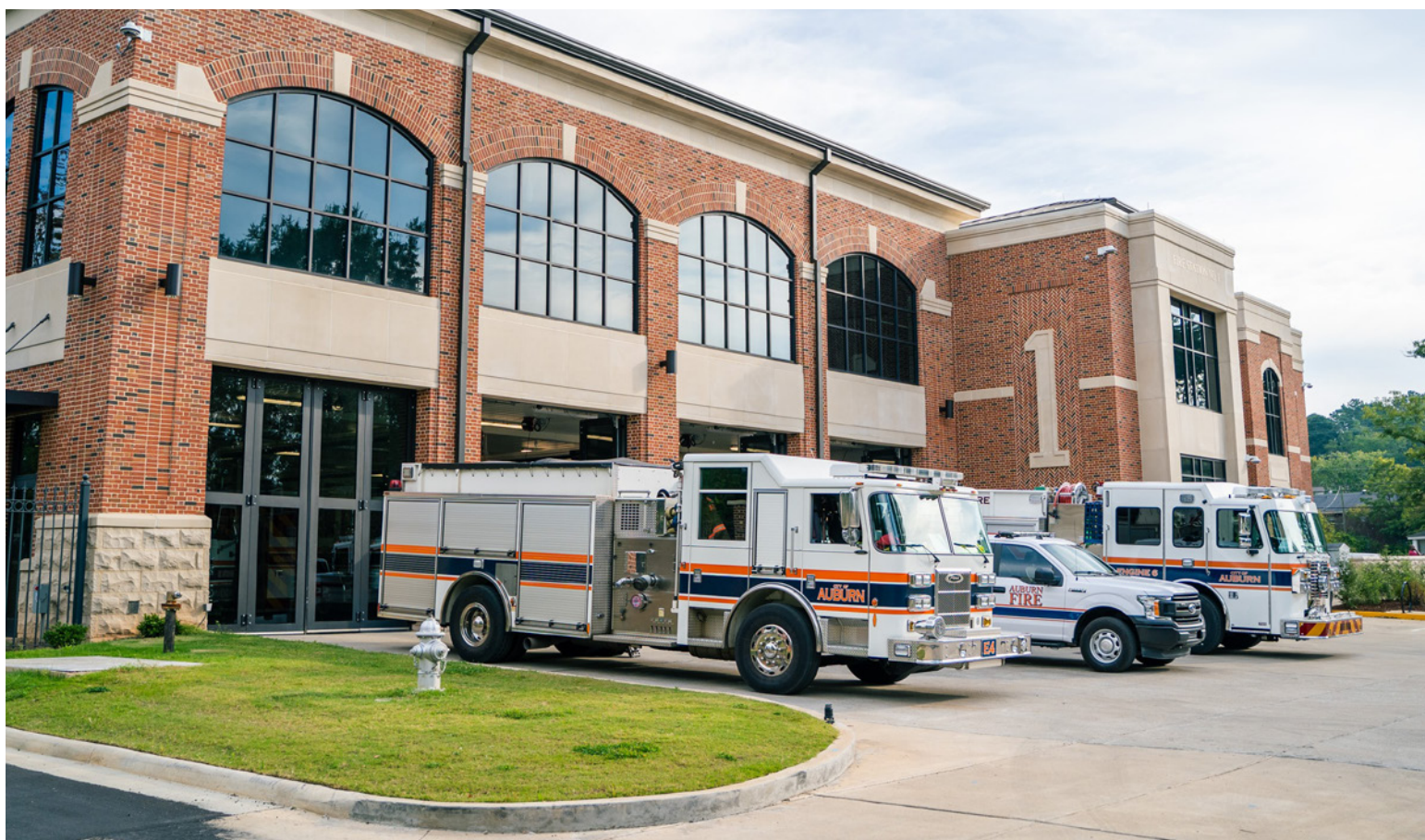
Auburn Fire Station 1
